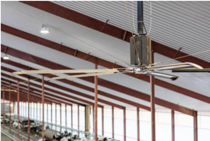
***"The building's aluminum-covered ceiling, which features six inches of insulation, works with the fans to help keep equipment and interior surfaces from freezing."***
